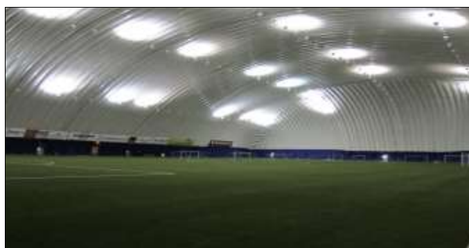
Fig 1: Interior of the air supported sport hall in Mo i Rana, Norway [16]
